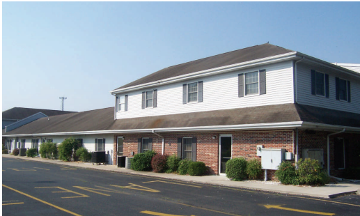
Community Legal Aid Society, Georgetown, DE Community based office facility
