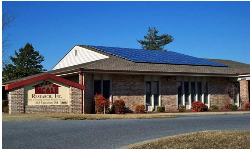
A successful installation of 66 solar photovoltaic panels on the south facing roof of NCALL's Dover office was completed in February. The goal is to reduce NCALL's electrical costs by 70% through actual generation and the sale of renewable energy credits. Utilities are always a variable operating budget item outside of one's control. Using a renewable energy source such as solar helps to stabilize energy costs, thus, reducing vulnerability.
